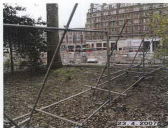
Effective fencing in position
