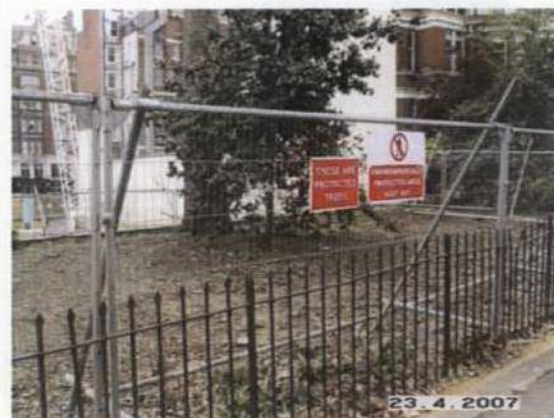
Fencing with signs
