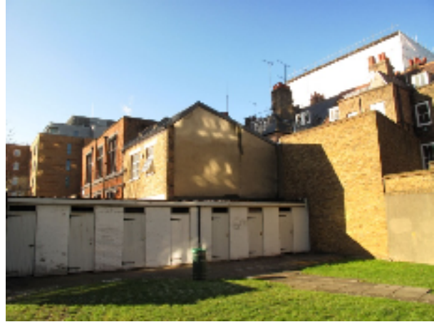
Existing side of the property (East)
