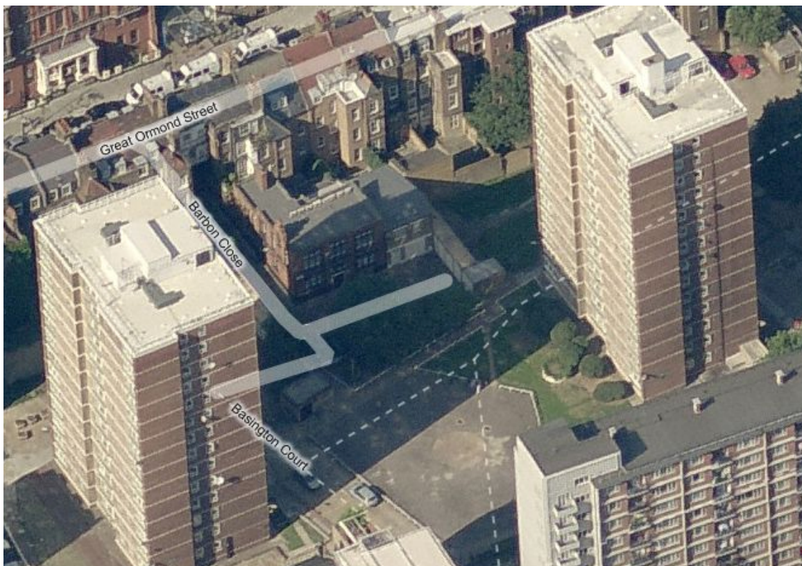
Existing ariel view of Barbon Close and immediate surrounds
