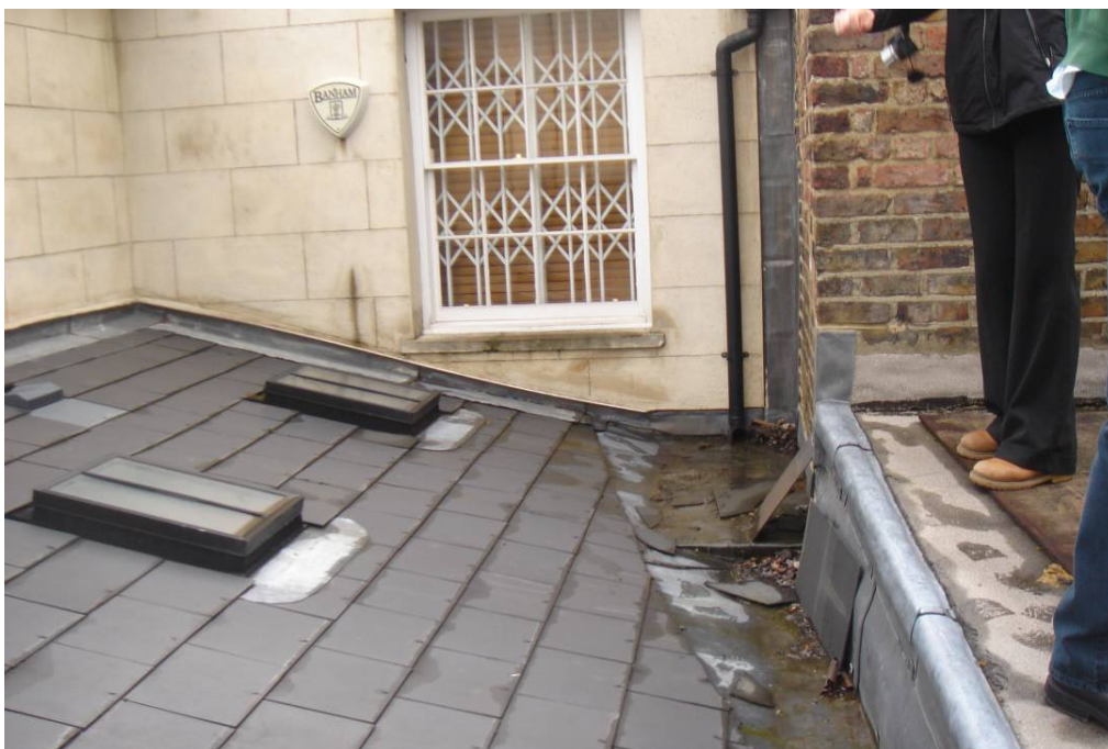
Low Pitched Rear Slate Roof Showing the valley gutter
