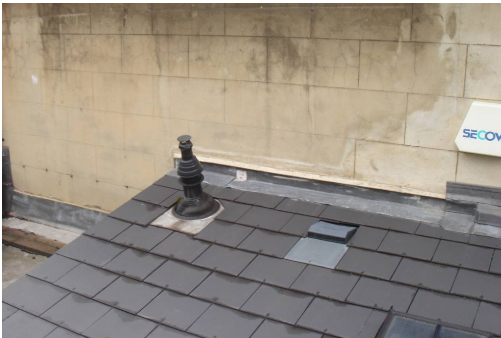
Low Pitched Rear Slate Roof (Showing Boiler Flue)
