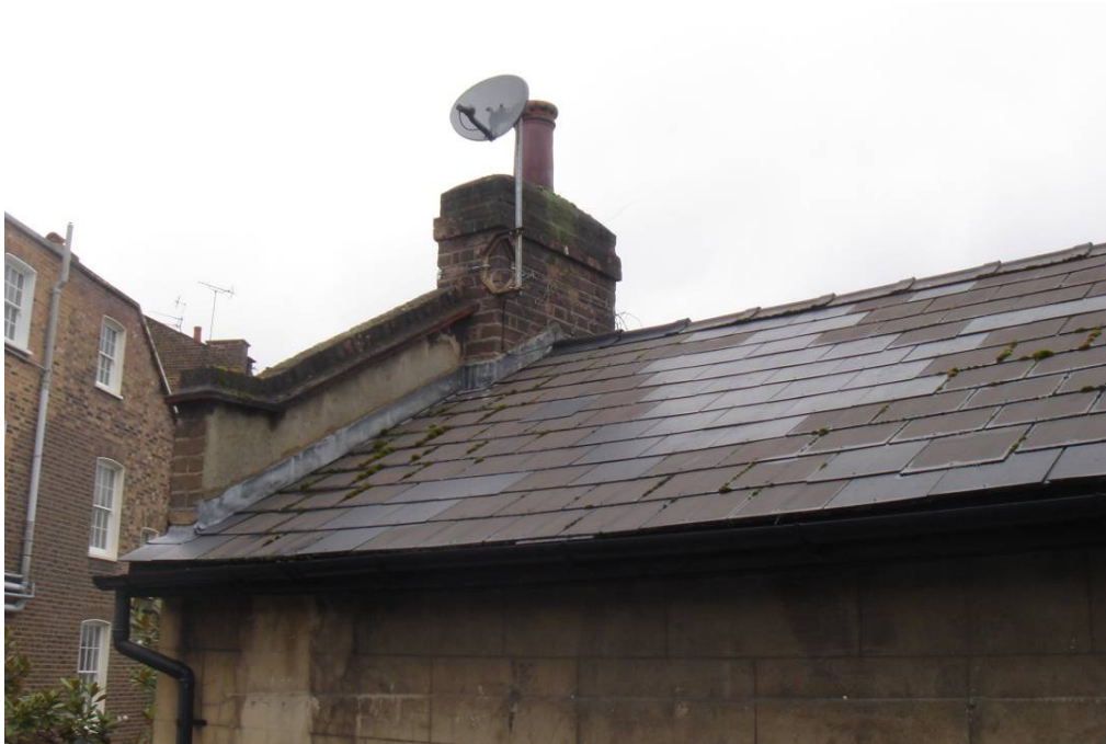
Rear End Gable Wall Parapet
