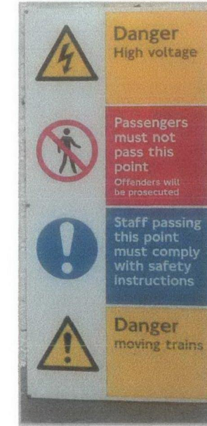
W1/4 - Existing No.102 end-of-platform warning wall-mounted to one side: to be retained
