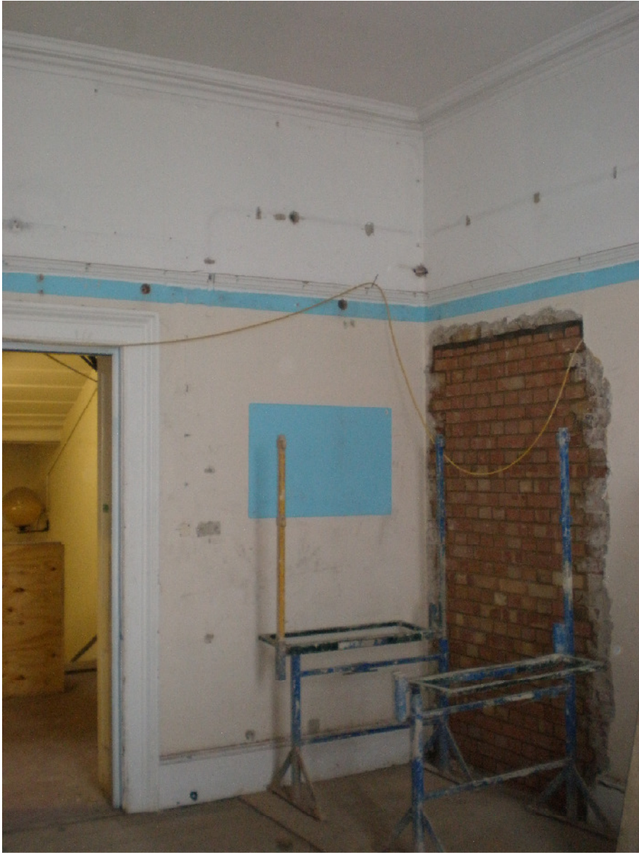
Second Floor Room 2/31
