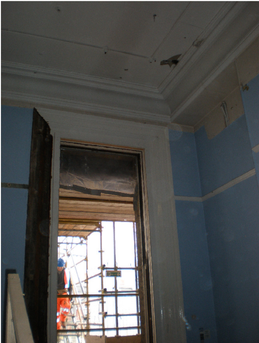
Room 1/08 - Window surround (left architrave temporarily removed)
