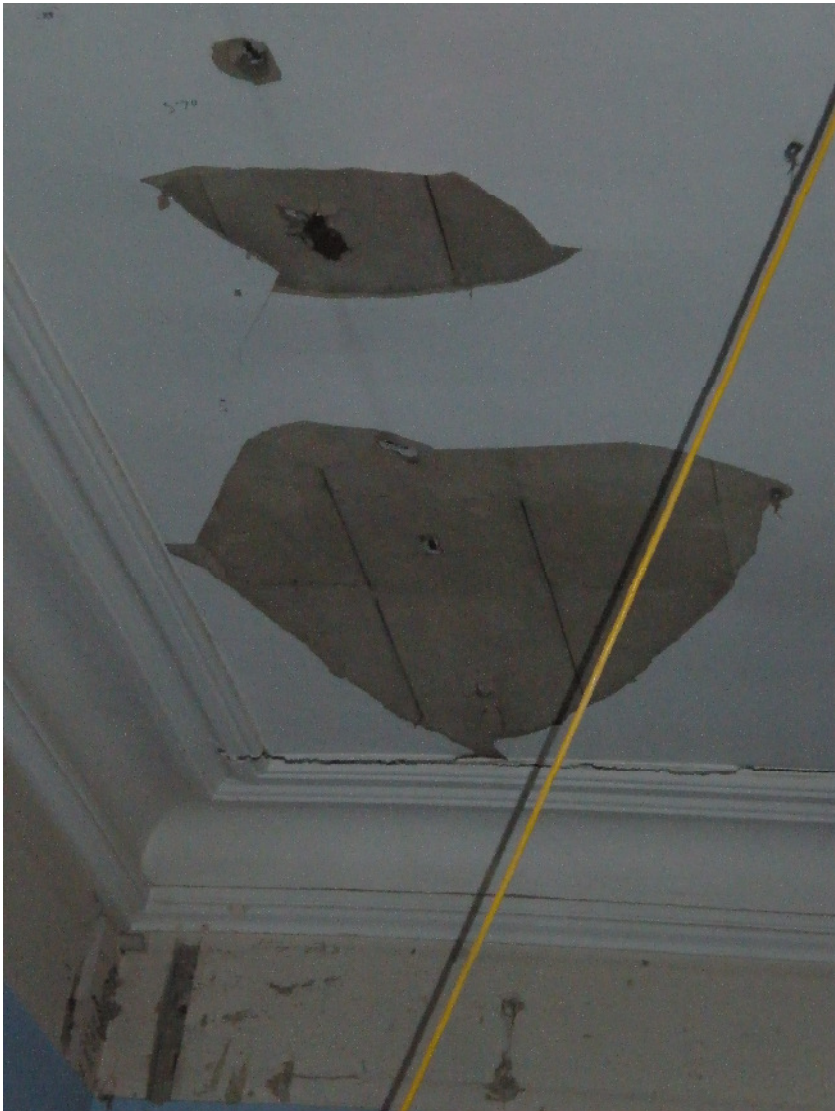
Room 1/08 - Central area of Ceiling showing modern plasterboard
