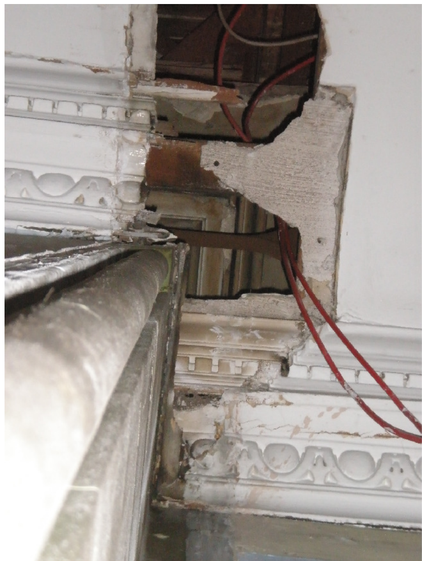
Original (higher) and later (lower) ceilings
