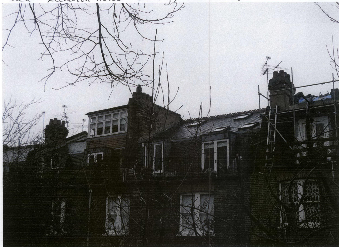
Roof/Loft conversion to No 160 Goldhurst Terrace NW6
