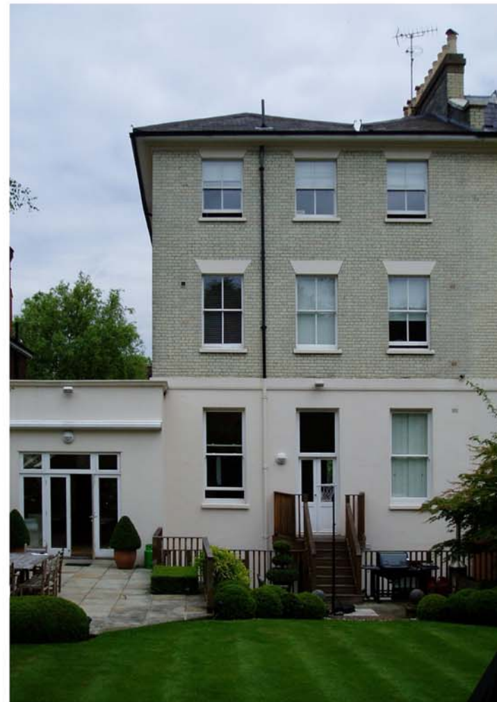
VIEW OF REAR ELEVATION
