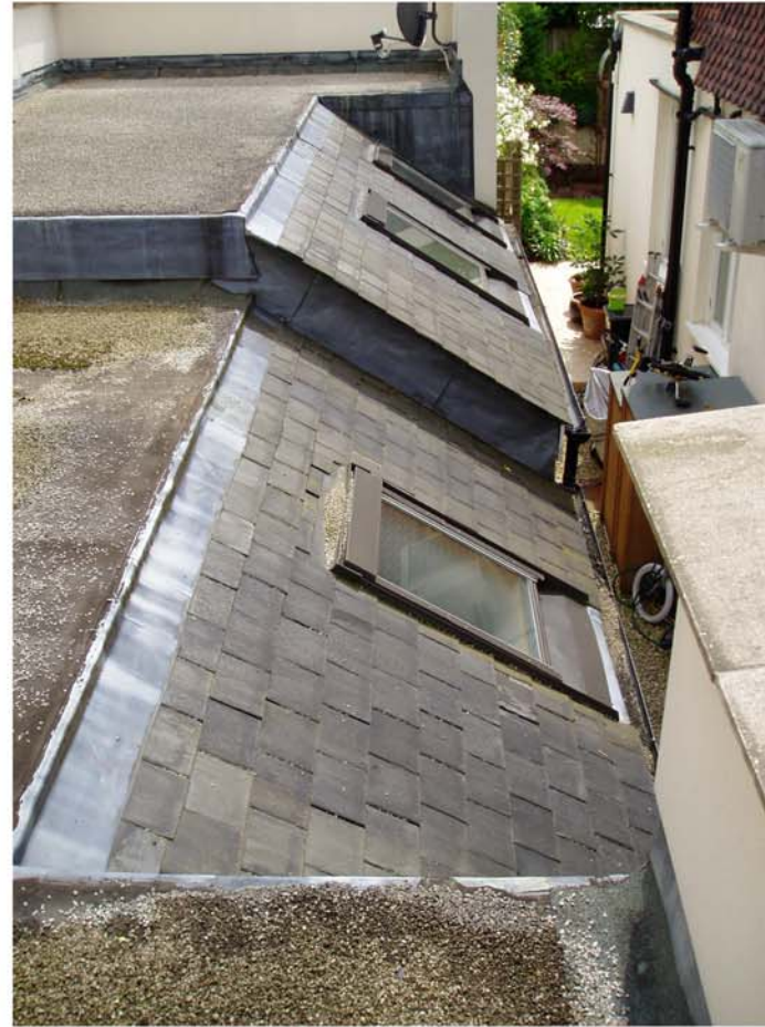
VIEW OF EXISTING ROOF TO EXTENSION
