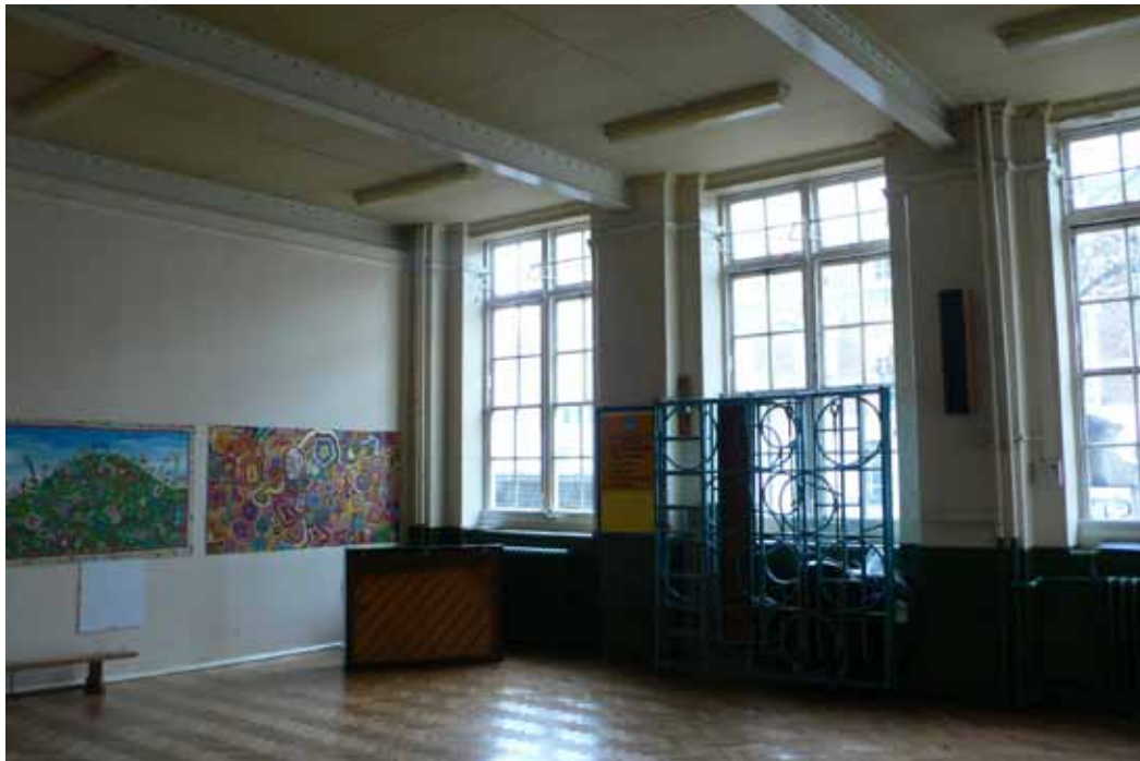
1. Existing Main Hall, looking east
