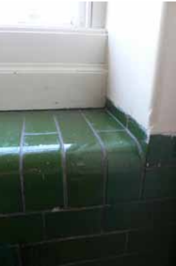
4. Existing Main Hall, Detail glazed brick dado
