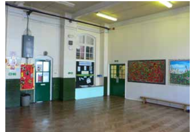
2. Existing Main Hall, looking south
