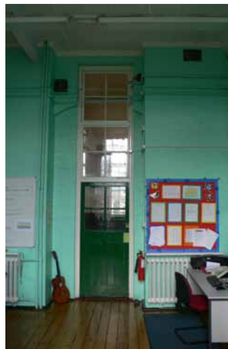
7. Existing staff room, looking north west
