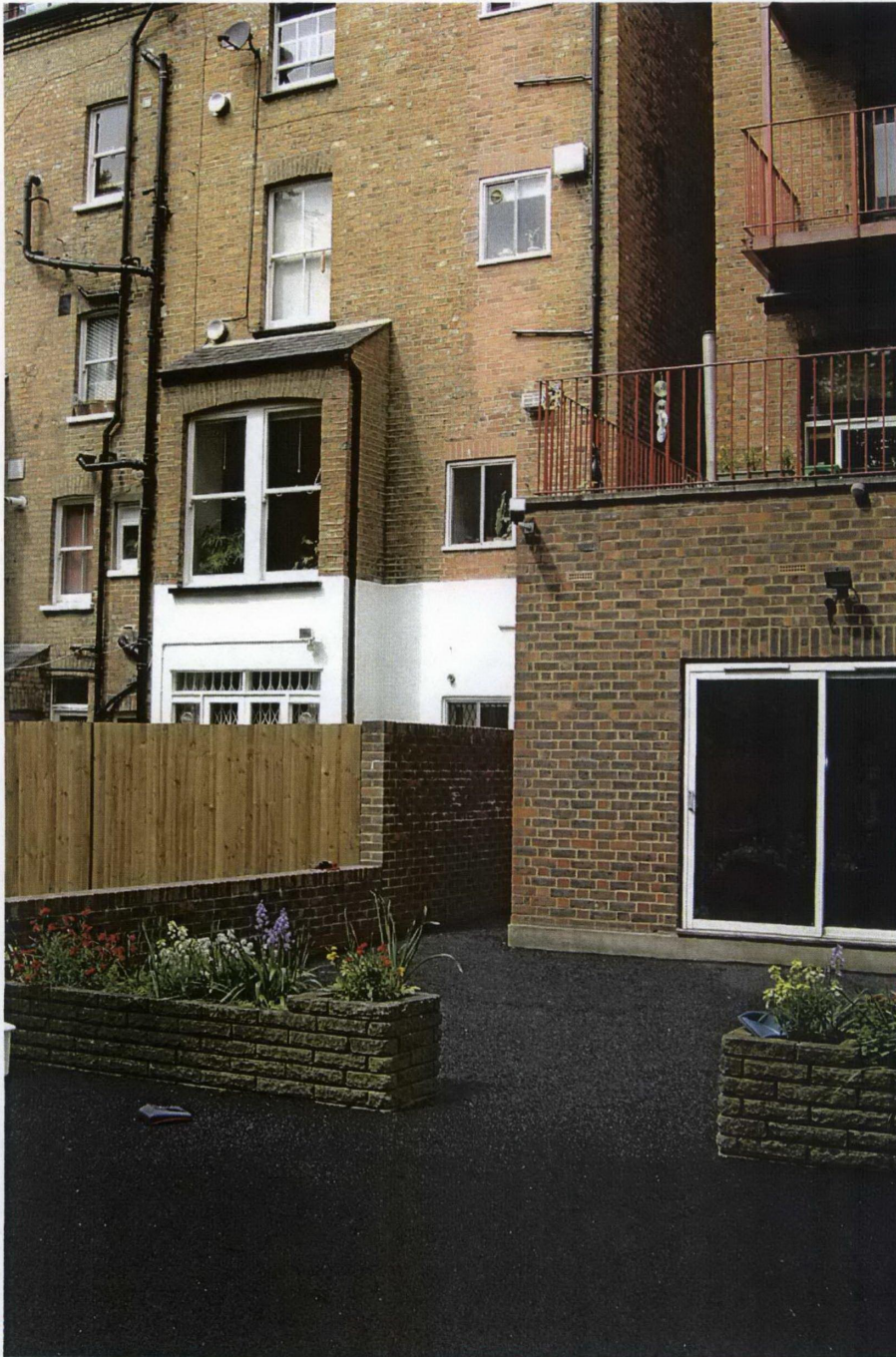
Fig.3 Rear elevation of 21 Greencroft Gardens shown in left side of photograph.
