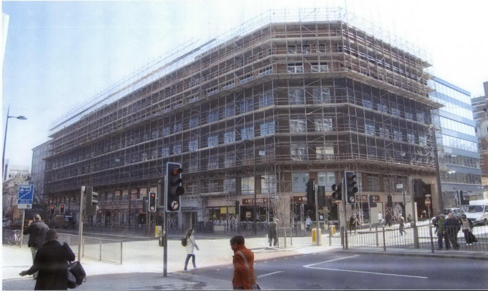
Clifton House, Euston Road – Photo Scaffold insitu - Drawing No. BSB/Eus/004
