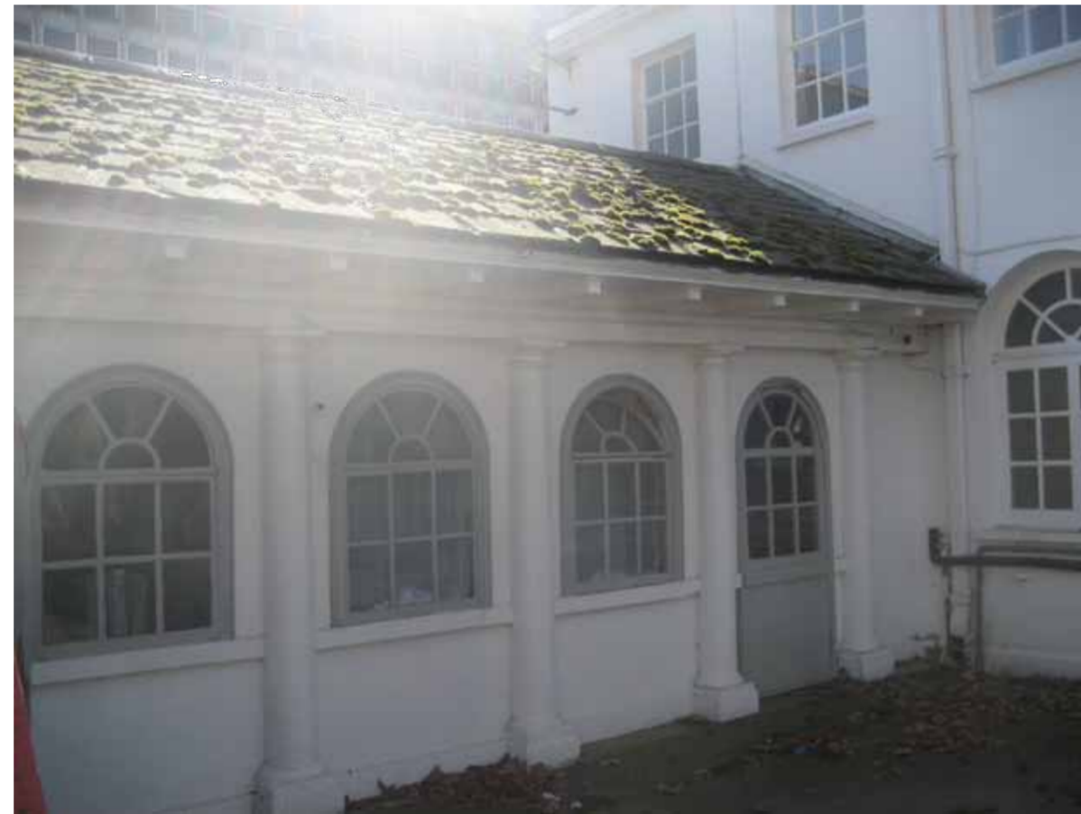
Photograph 8 - External view of Small Nursery
