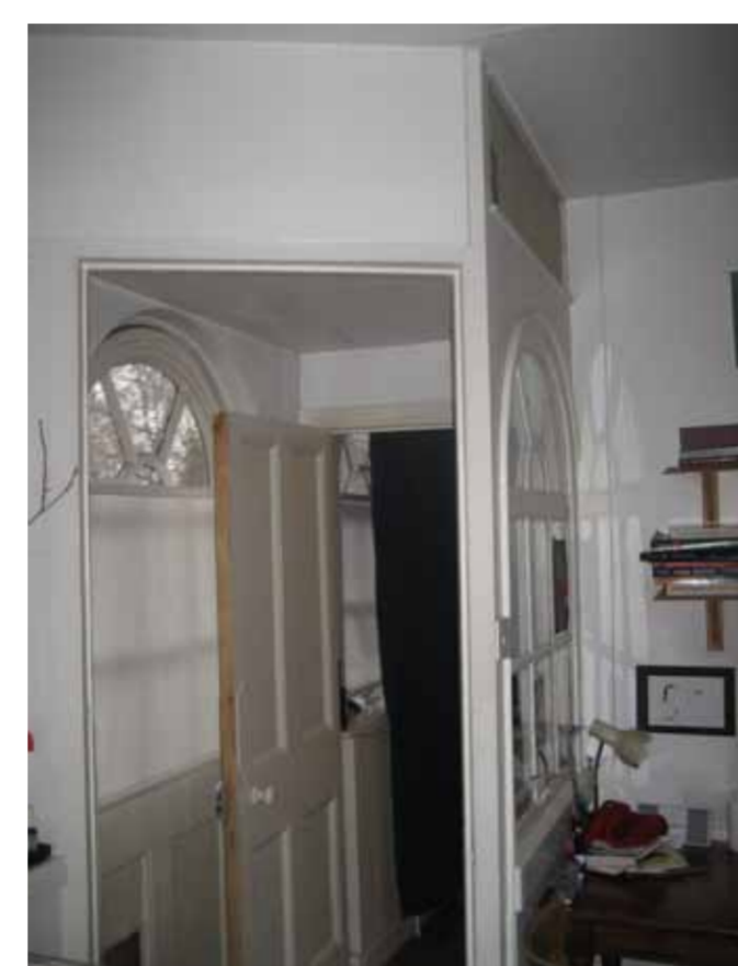
Photograph 14 - Internal view of the Lodge
