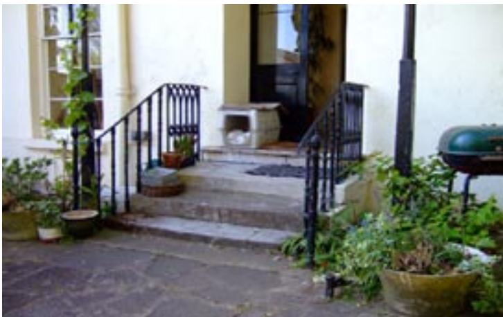
Existing rear patio
