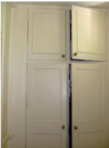
Existing entrance modern cupboards
