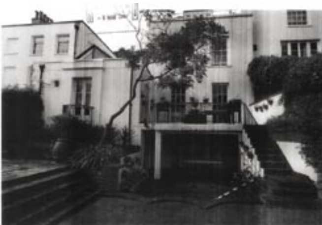
No.83 HIGHGATE WEST HILL, drawings and photo before works. Application No: 2007/1215/L, L2007/1212P
