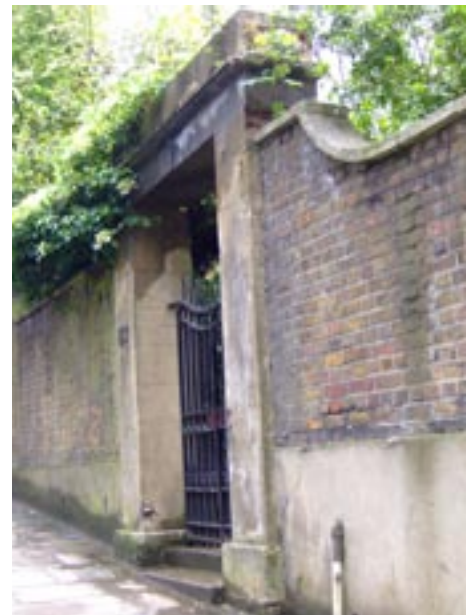
Existing entrance portal
