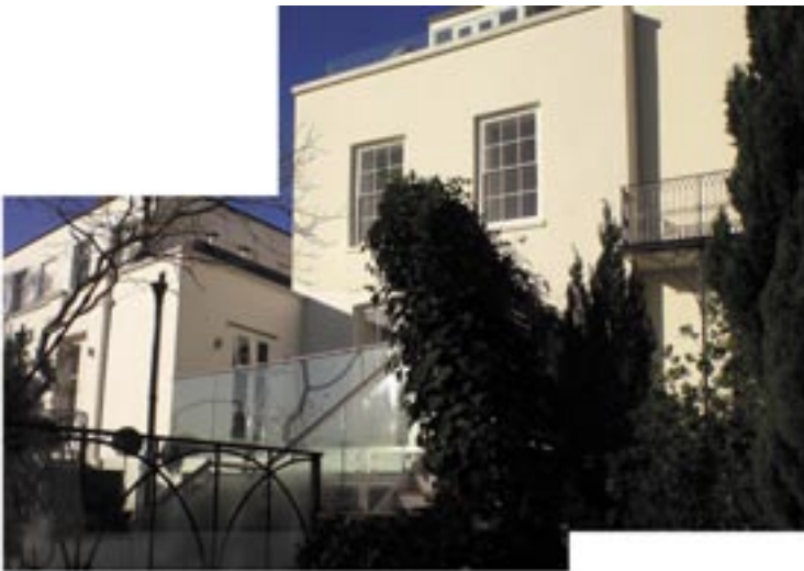
No.83 HIGHGATE WEST HILL, Proposed drawings and rear elevation photo after works. Application No: 2008/5158/P, 2008/5352/L.
