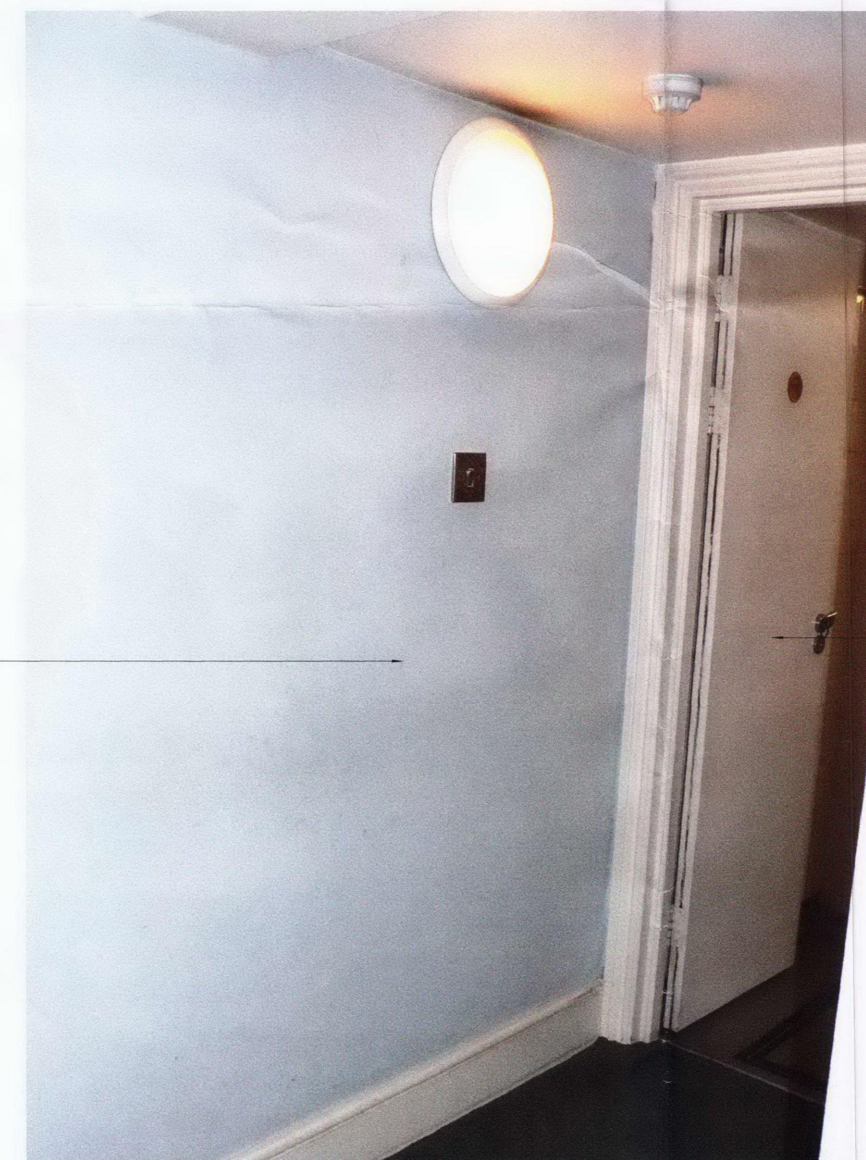
03 BASEMENT FLOOR VIEW - LOBBY B29 A0229 EXISTING
