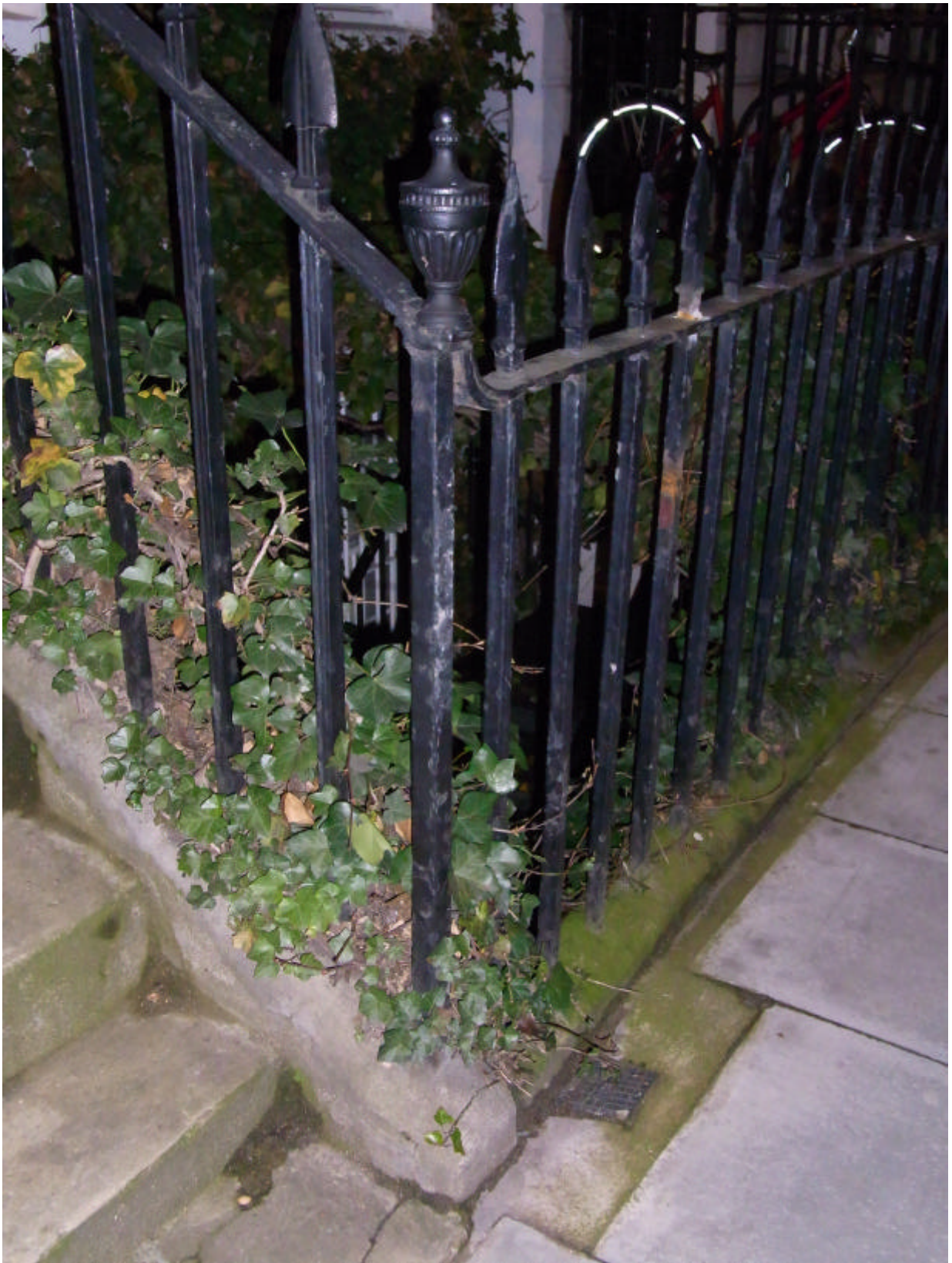
6. Examples of railings from no.91 Judd St, of which proposed railings will match.
