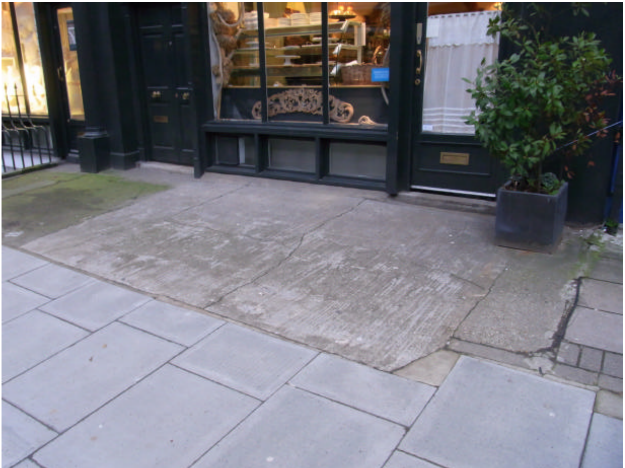
4. Existing entrance to coffee shop with concrete forecourt.
