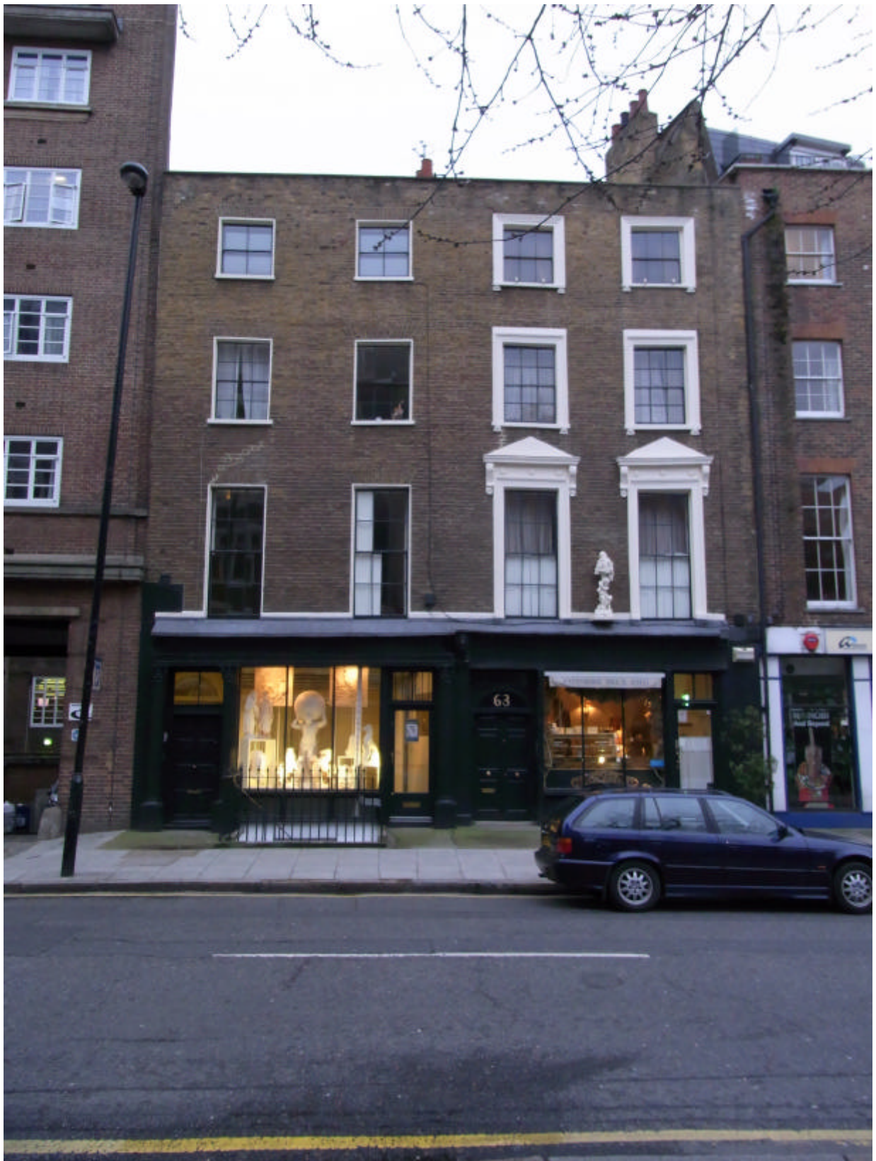
3. View from Judd Street of no.63 on the right and no.61 on the left.
