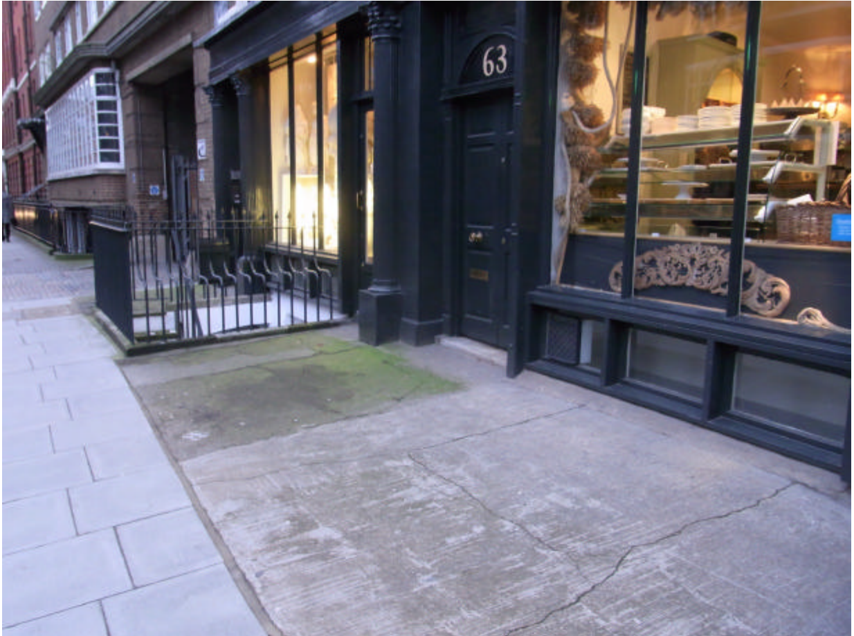
5. Concrete forecourt set forward slightly from stone base of no.61.
