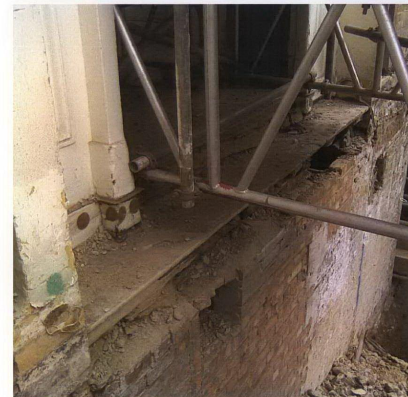
Northern Office Entrance, existing York Stone threshold.
