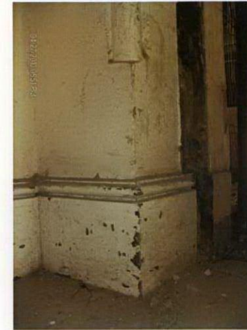
Northern Office Entrance, Existing timber skirting.
