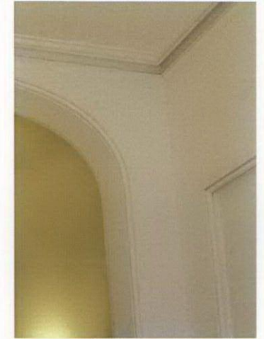
Northern Office Entrance, decorative finishes
