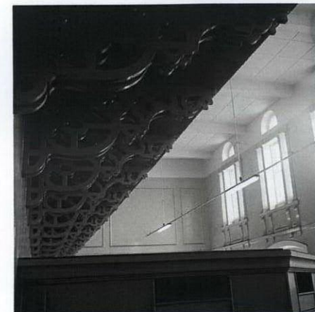
Cast-Iron brackets for first floor balcony
