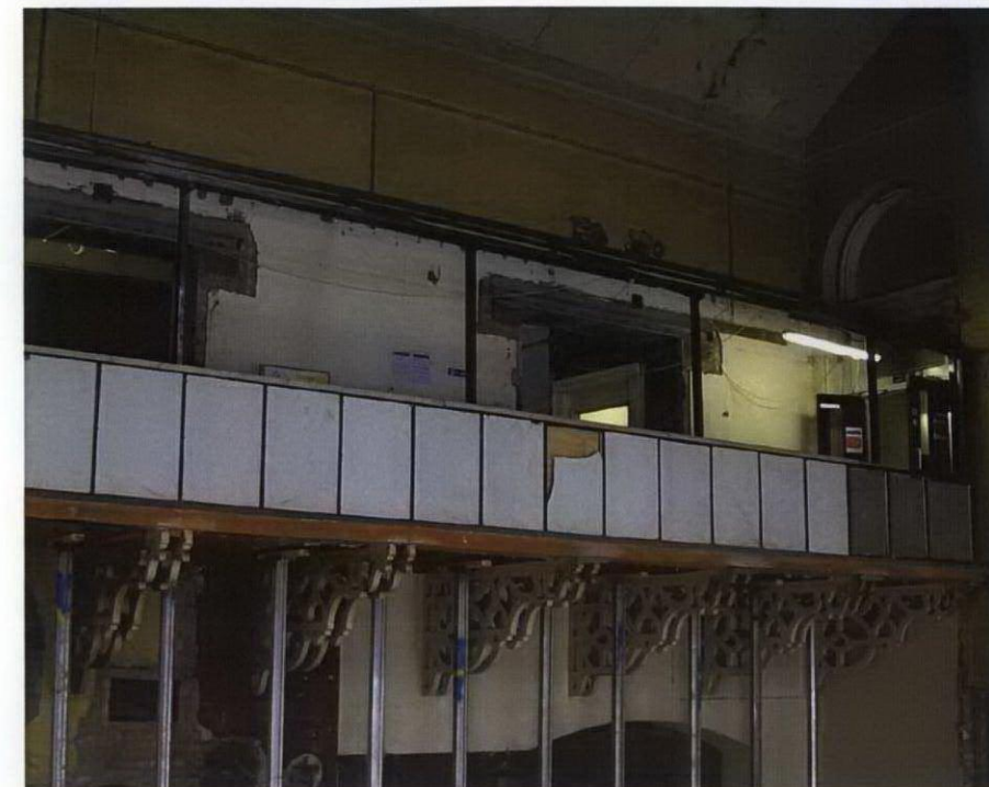
First floor mezzanine link and cast iron brackets.
