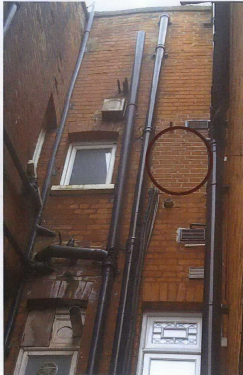
EXISTING WINDOW INFILLED
