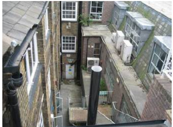
3 VIEW OF LIGHTWELL SHOWING No 14 PARKWAY
