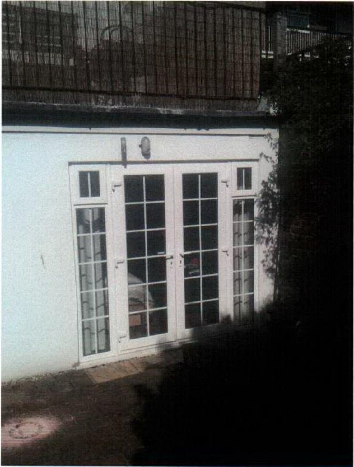
GROUND FLOOR DOUBLE DOORS LOCATED BELOW THE TERRACE.
