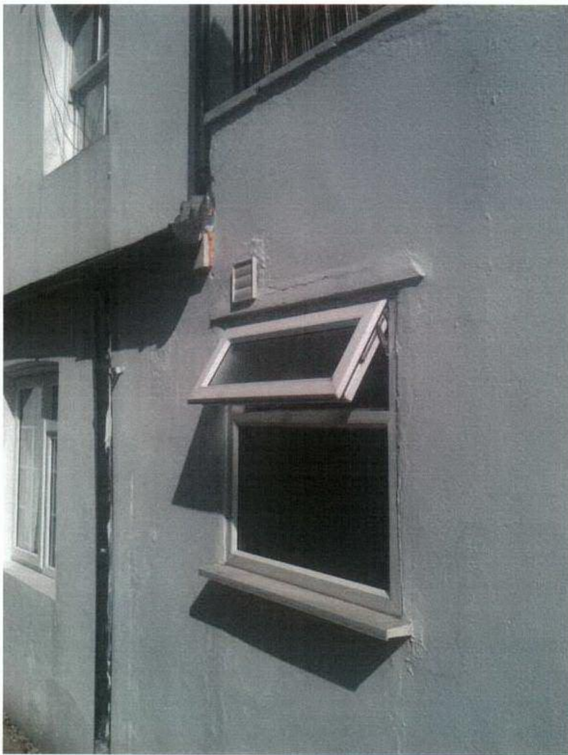
PASTING WINDOWS ON THE GROUND FLOOR EXTENSION.
