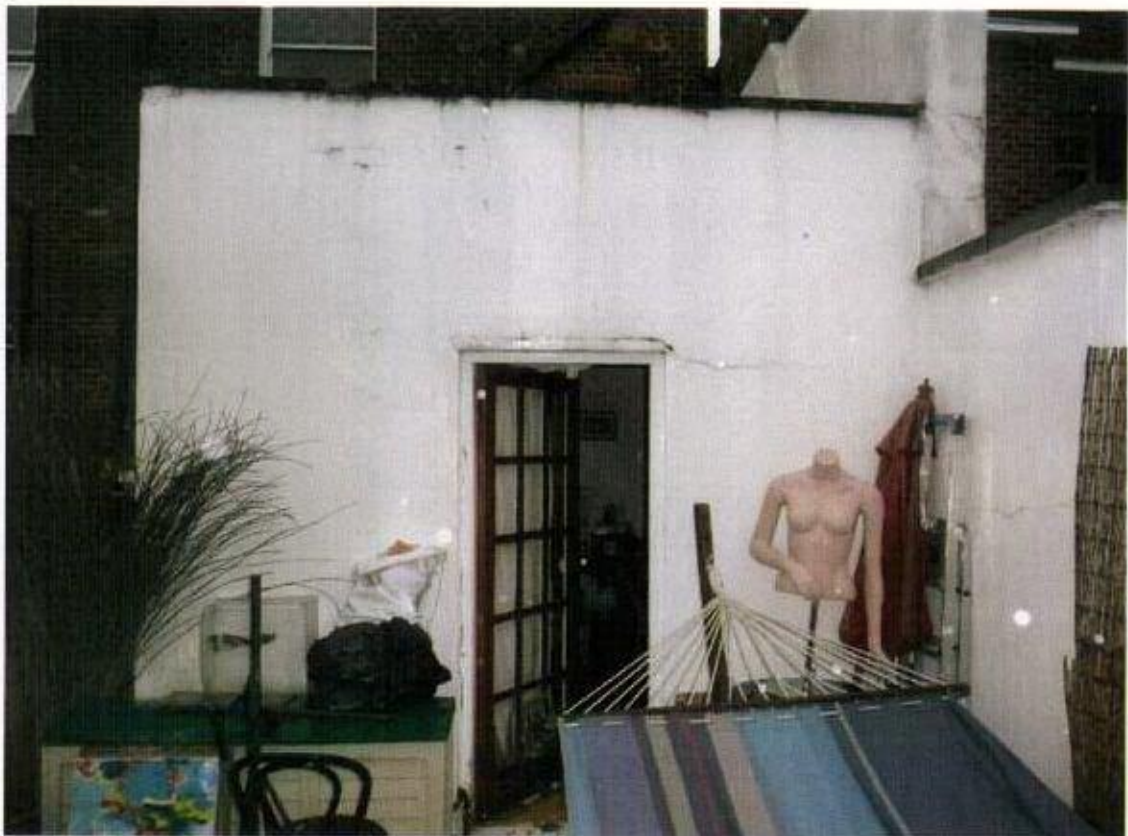
EXISTING REAR ELEVATION + DOOR PROVIDING ACCESS TO THE TERRACE.
