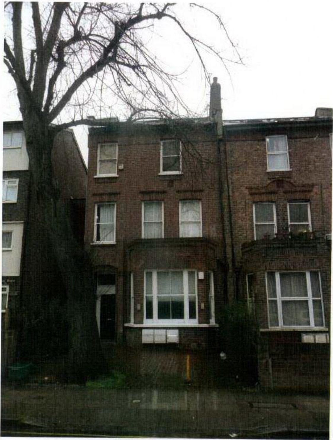
THE FRONT OF 121 GOLDHURST TERRACE.
