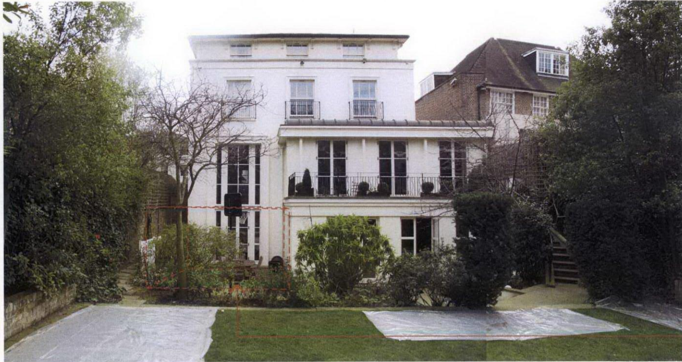
1 Existing North Elevation (Site visit May 2010)
