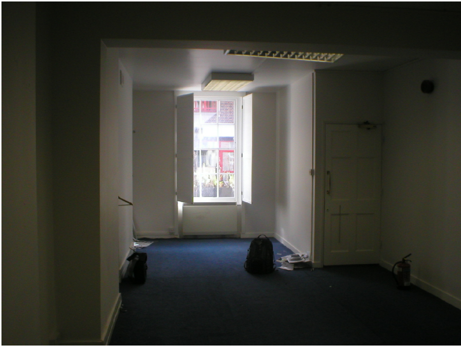
Photograph 1 - Existing Ground Floor Interior, Front
