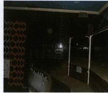
1900 balcony with 1960 tiles behind
