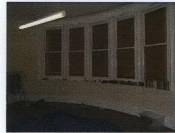
West wall, with windows currently boarded up
