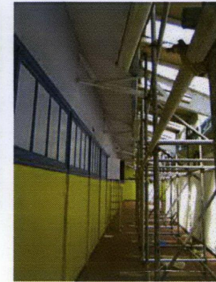
Corridor Looking North
