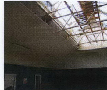
Modern suspended ceiling, with original truss above.
