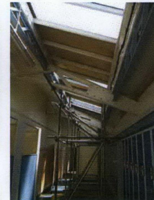
Original roof structure
