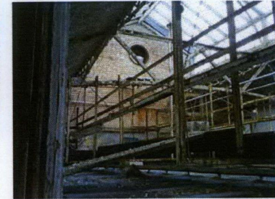
Space above 1960 suspended ceiling
