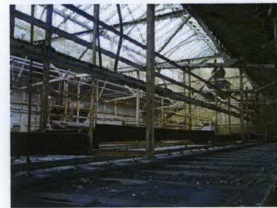
Space above 1960 suspended ceiling
