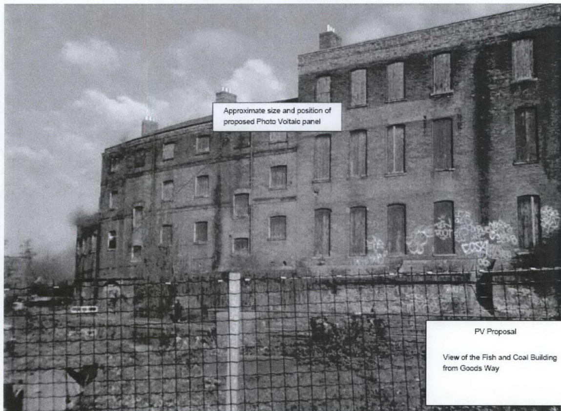
Figure 2: Photo showing proposed location of PV panel
