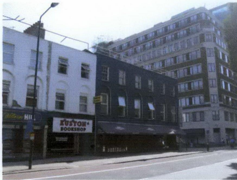
View of the black rendered façade of 34-38 Eversholt Street with the 9 storey Euston House in the background.
