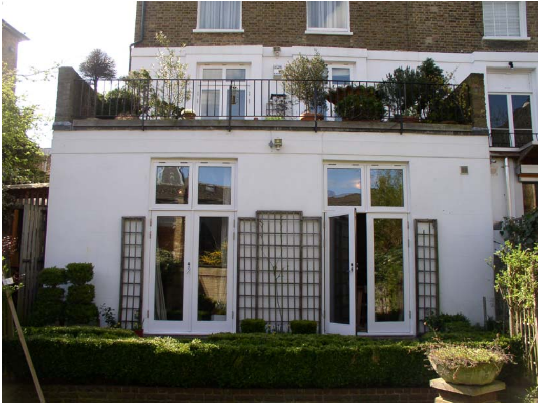
Photo No. 1 Rear elevation
