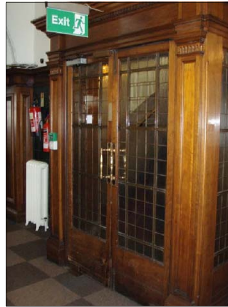
P01 PHOTOGRAPH OFFICE ENTRANCE DOORS
