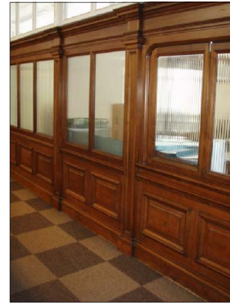
P02 PHOTOGRAPH TIMBER PARTITIONS TO SMALL OFFICES
