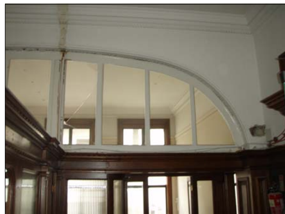
P08 PHOTOGRAPH VIEW OF ELEVATION ABOVE FROM OPPOSITE SIDE
