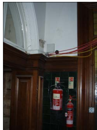
P09 PHOTOGRAPH PLASTER MOULDING TO UNDERSIDE OF ARCH OBSCURED BY HIGH LEVEL TIMBER FRAMING
