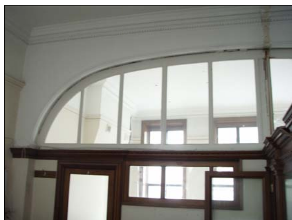
P07 PHOTOGRAPH VIEW OF ELEVATION ABOVE FROM OPPOSITE SIDE
