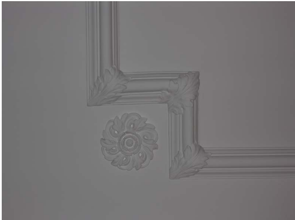
Fig 13 Detail of plaster ceiling decoration in room 28 (2873.jpg)
