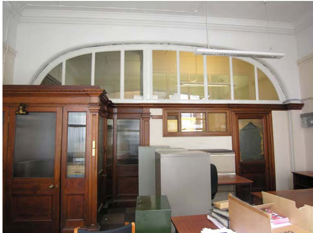
Fig 7 North wall of room 2. To the left, a 2-leaf door to the central passage; to the centre and right, a wall separating room 2 from room 12, with glazing above it. (2777.jpg).
