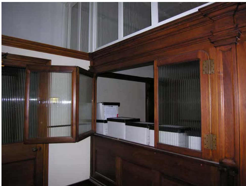
Fig 9 Folding 3-leaf window and counter in the east wall of room 16, internal face, looking north-east. A shelf or counter formerly under the window opening has been removed. (2876.jpg).
