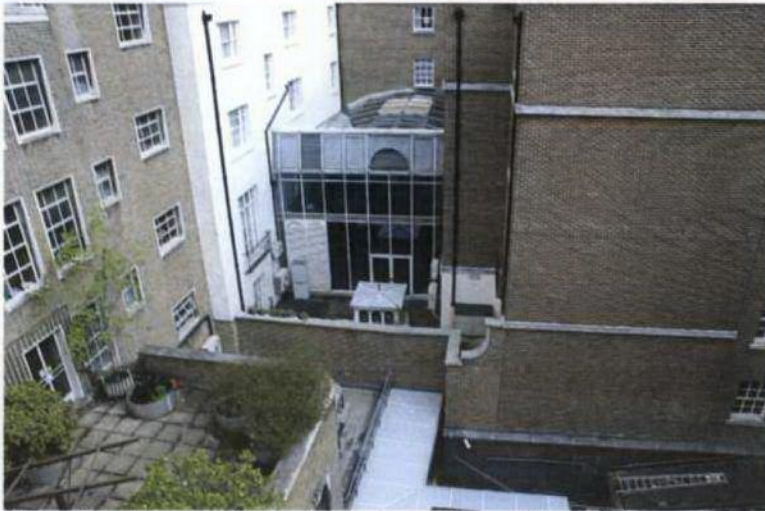
View of service yard (bottom) from upper floor of the Building
