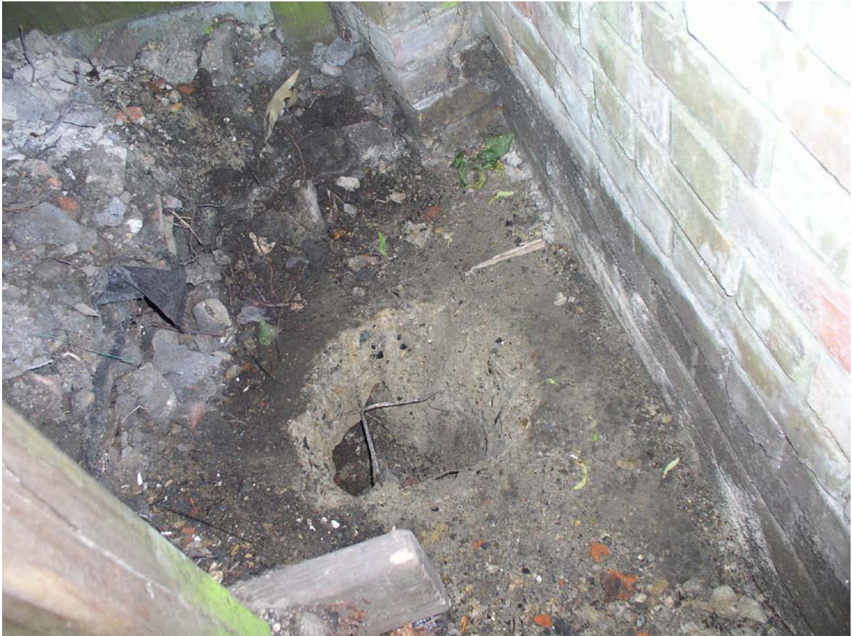
Photo No. 6 Trial hole at the rear where concrete slab was discovered.
