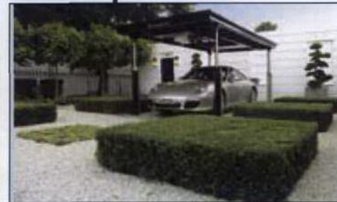
Any water finding its way into the Cardok is automatically pumped away.
