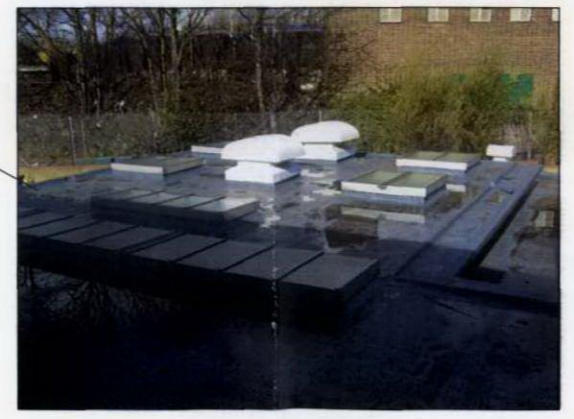
ROOF AREA FOR PROPOSED VENTILATION PLANT
