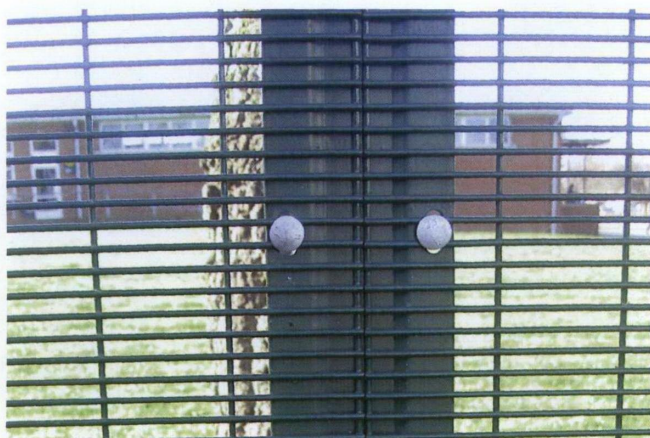
Securus flat panel system detail
