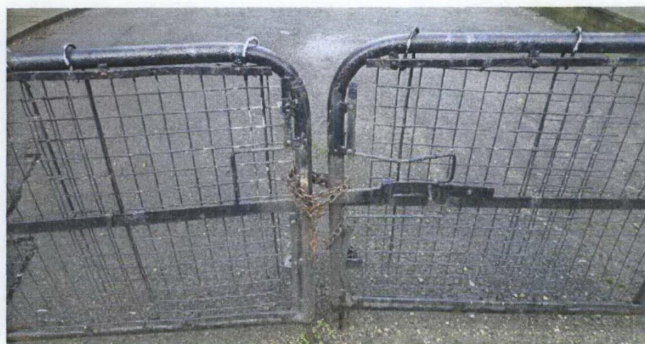
Existing metal gates are in poor condition
