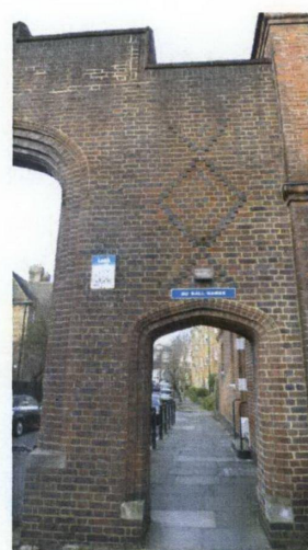
Brick arch detail showing tudor style arch and brick ornament diamond pattern
