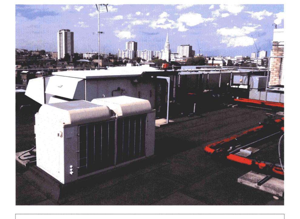
PHOTO H: View of smaller condenser and air handling unit on roof of 51-53 Hatton Gardens – looking North.
