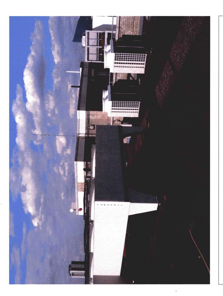
PHOTO C: Roof view showing the Van Spall condenser and two smaller Daikin condensers.
