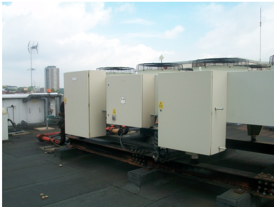
Figure 1.2b – (South West Facing) Photograph of existing dry cooler unit to be replaced by heat pump system.
