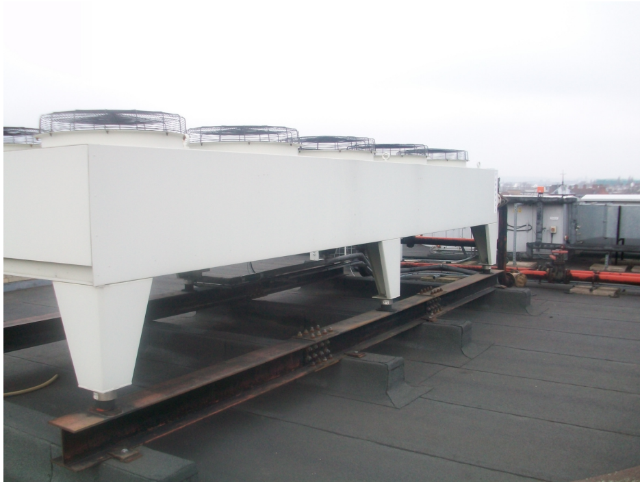
Figure 1.2a – (South East Facing) Photograph of existing dry cooler unit to be replaced by heat pump system.
