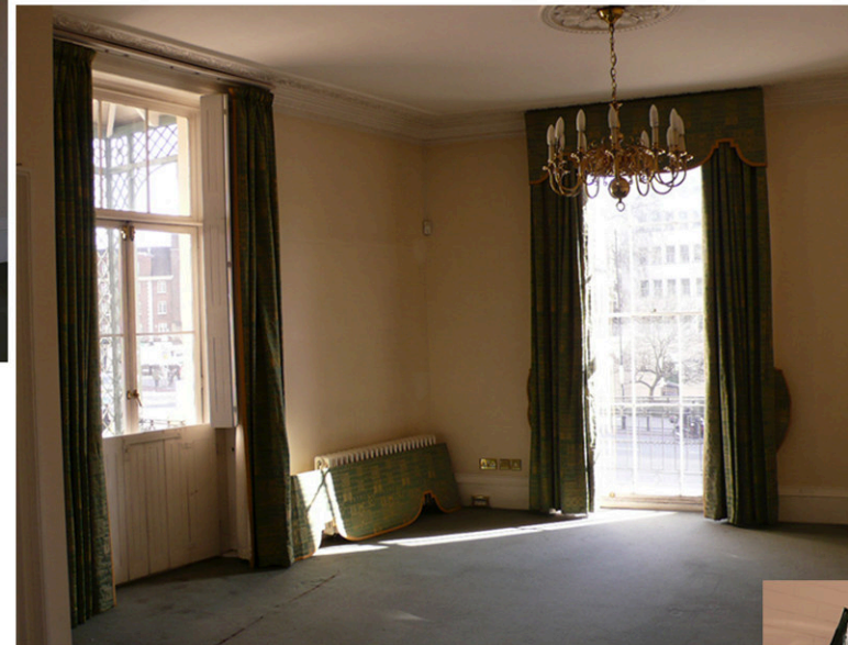
First Floor: Reception
