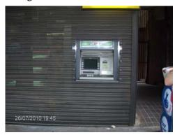
The existing roller shutter has been modified to give access to the ATM during the closed hours of the shop. An aperture was formed in the shutter curtain.
