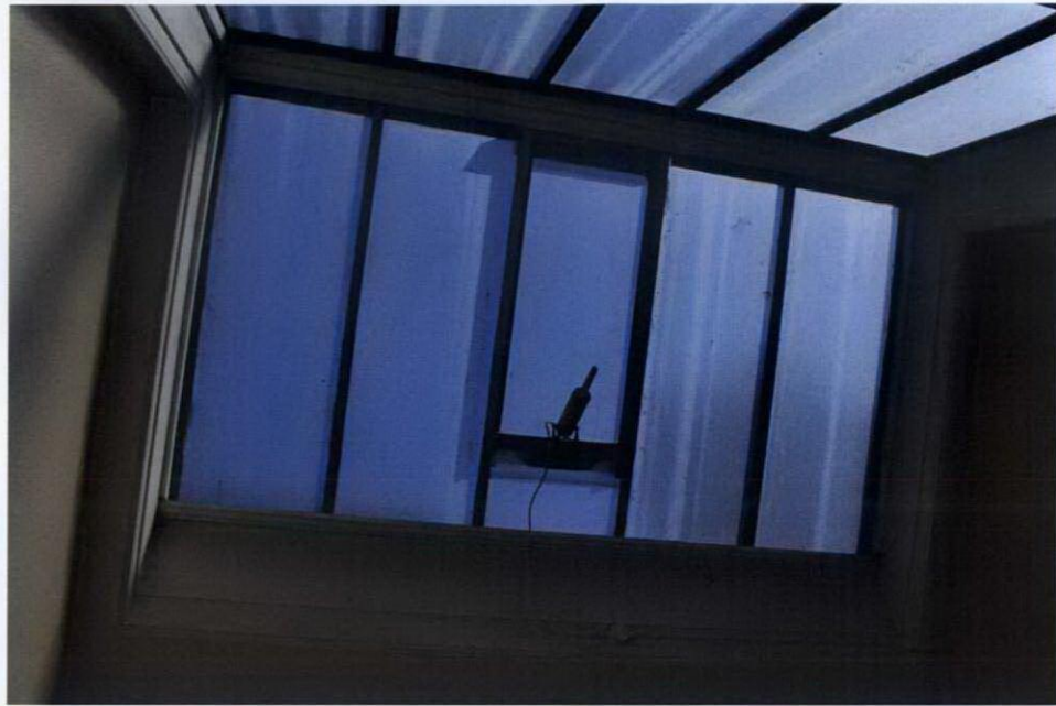
Skylight over staircase
