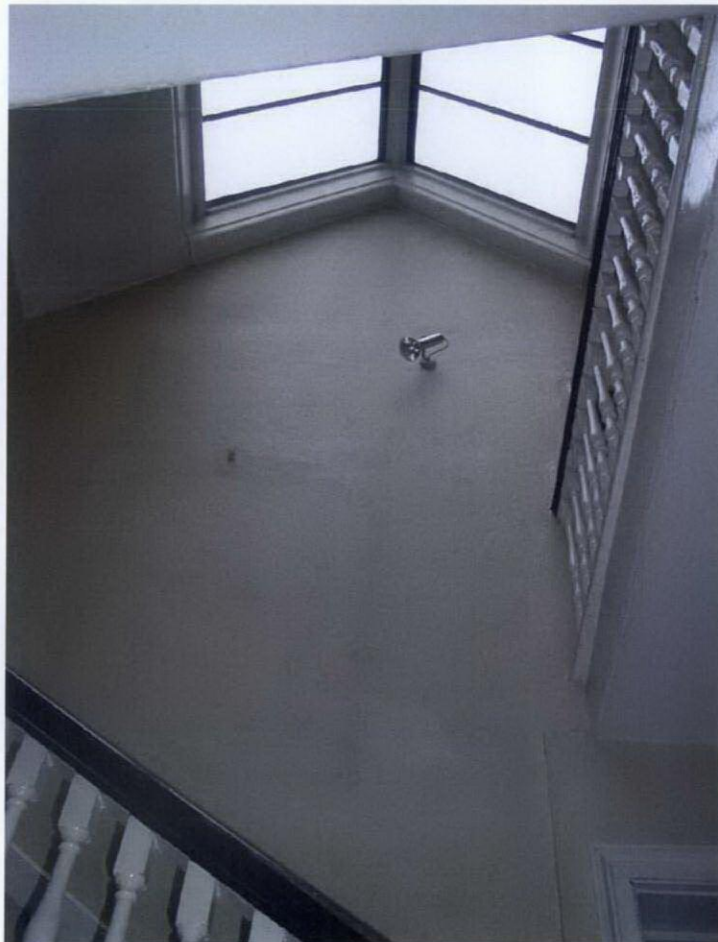
Stair landing at 3rd floor
