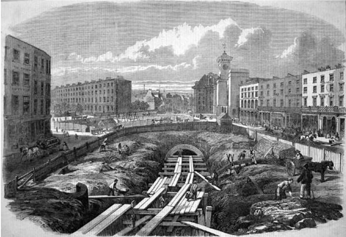
Figure 15: Construction of the Metropolitan Railway
