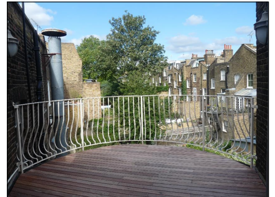
New railing and timber decking
