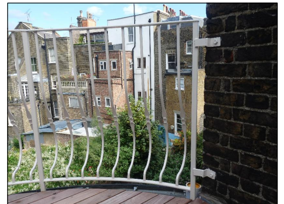
New railing and timber decking
