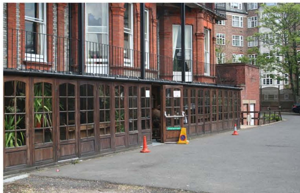
South (Rear) Elevation showing new Conservatory
