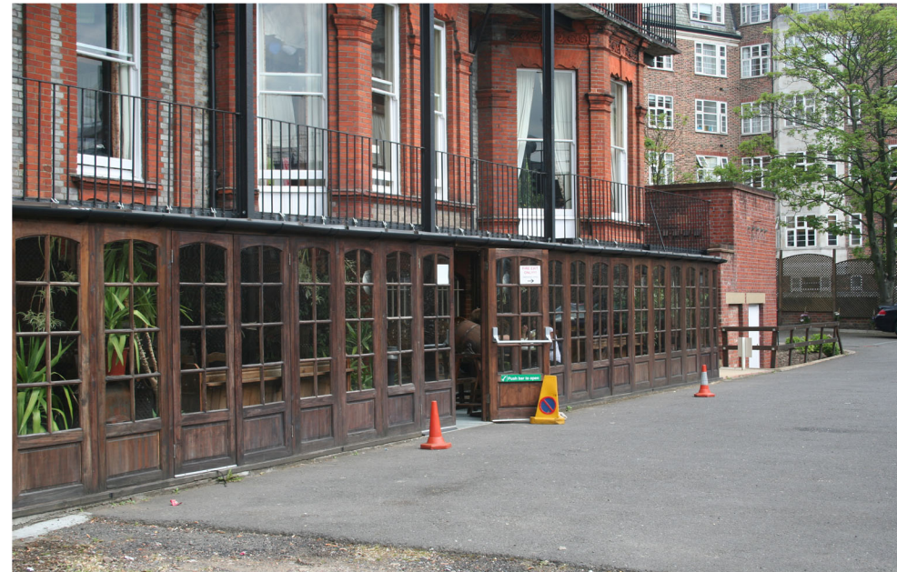
South (Rear) Elevation showing new Conservatory
