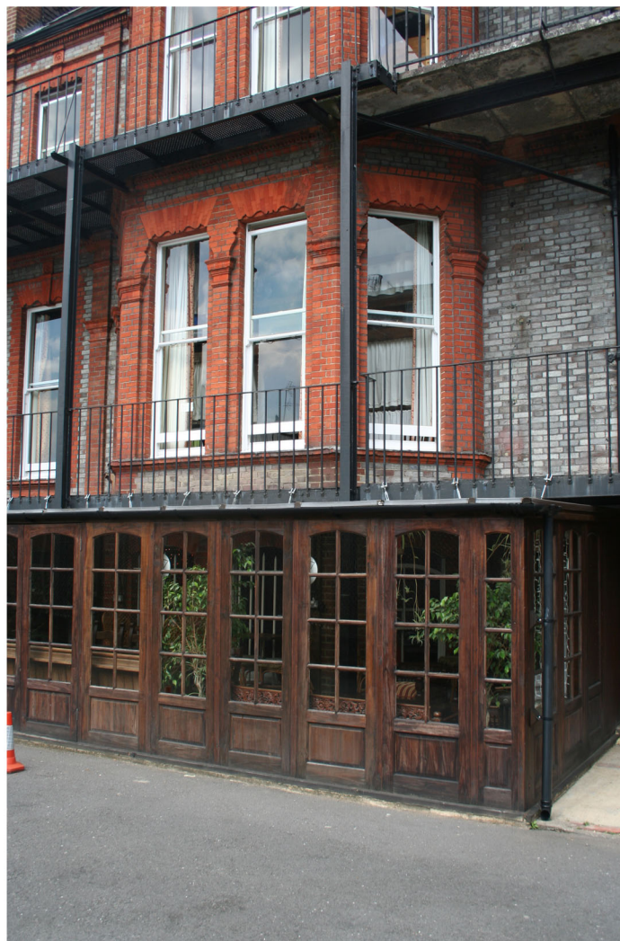
New Conservatory located under existing Fire Escape
