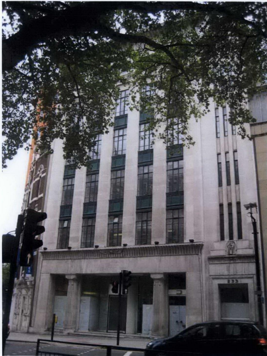
233 Shaftesbury Avenue Shaftesbury Avenue Elevation
