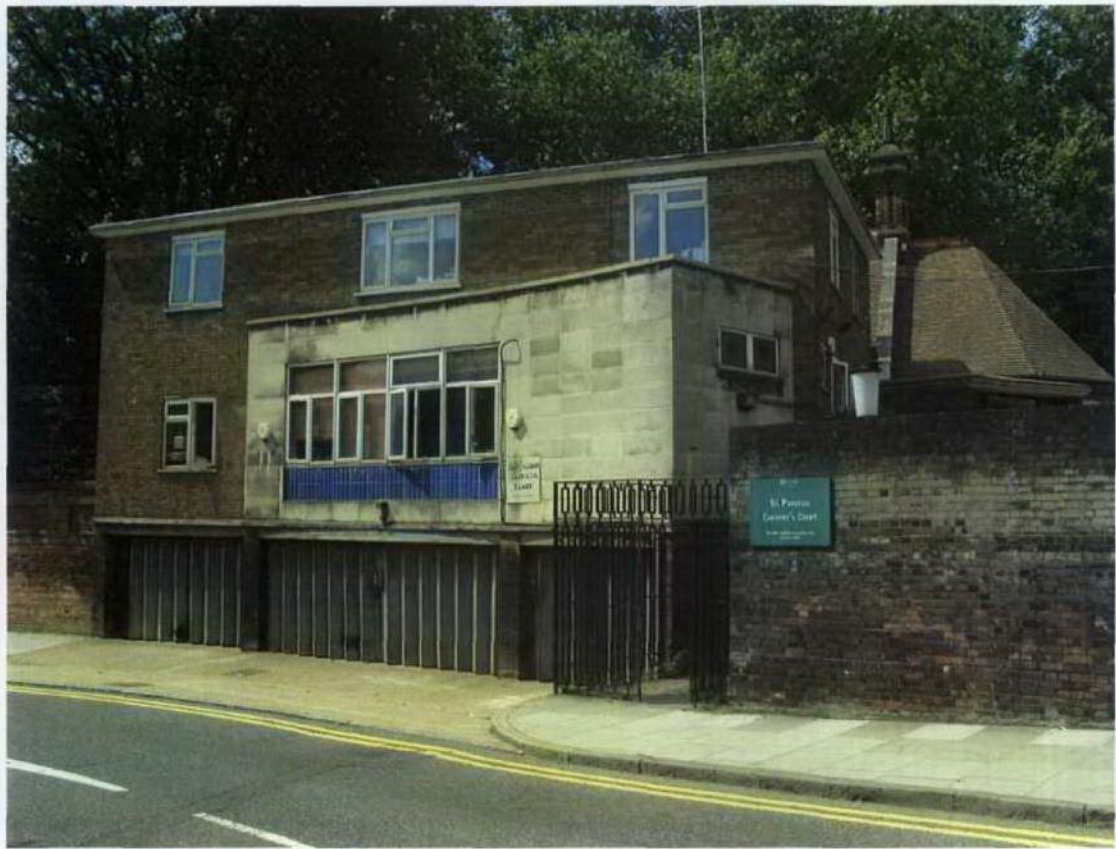
Fig 3 - View from Camley Street of 1950/60s addition
