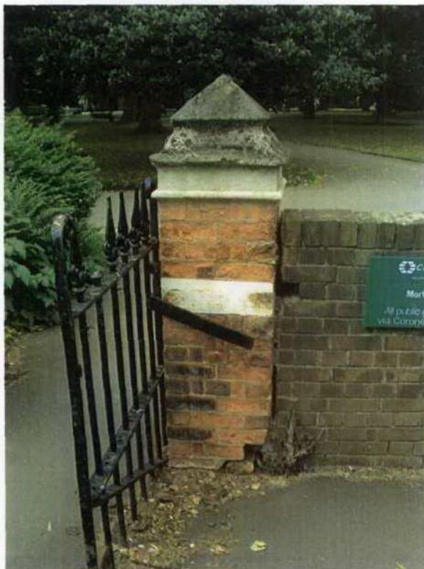
Fig 2 - Proposed Garden wall pier to be rebuilt
