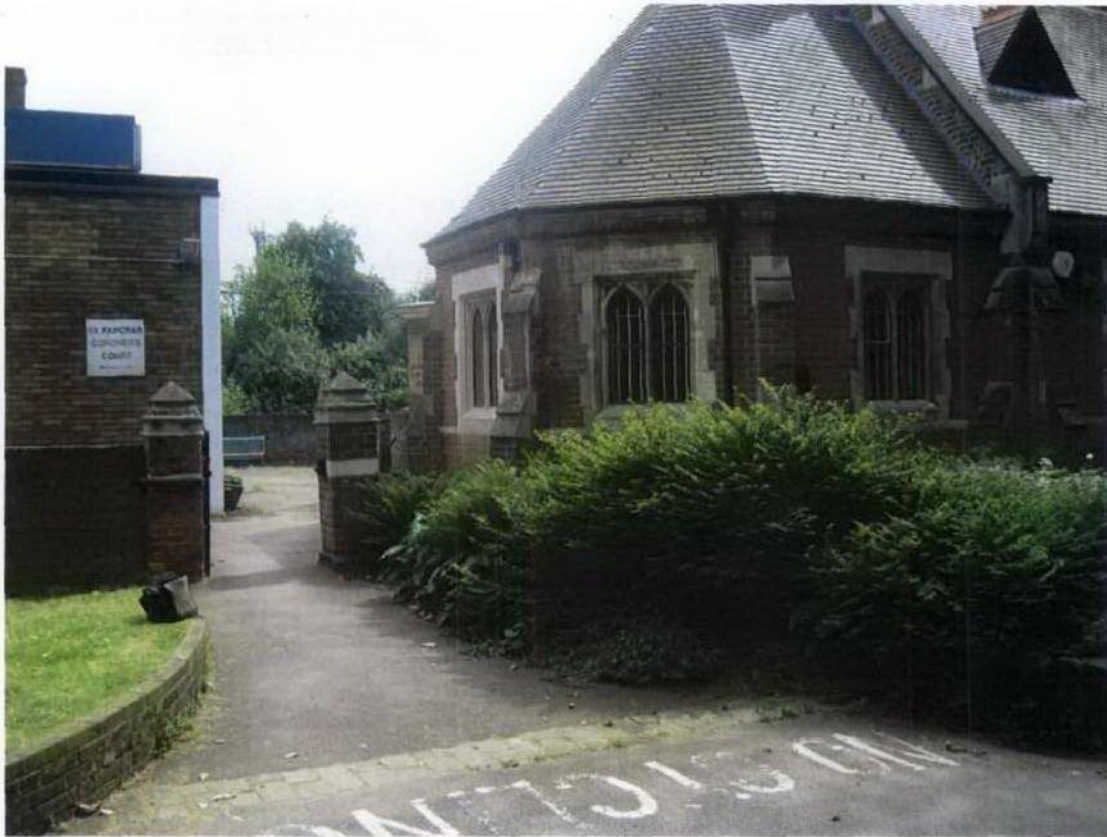
Fig 1 - View of external area between Court and Mortuary
