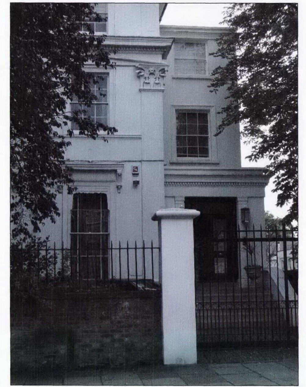
Side Addition at No.34
